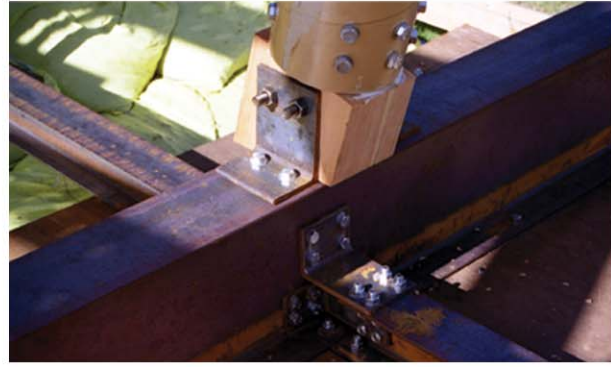
joints between steel beam and papertube
