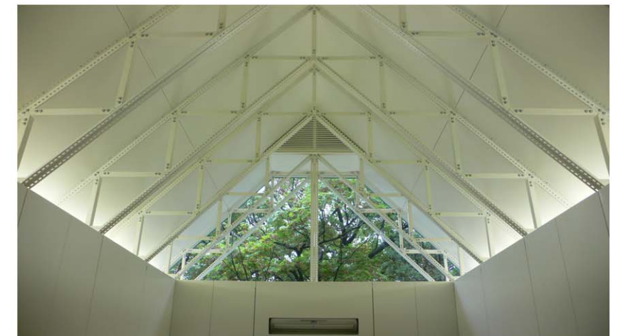
frame structure of the ceiling
