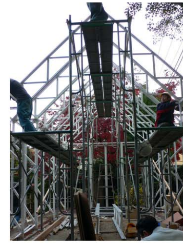
assembling on site
