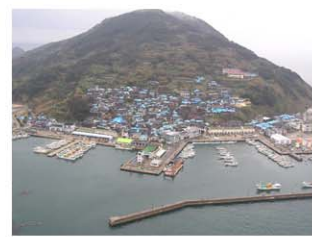
aerial view after the quake
