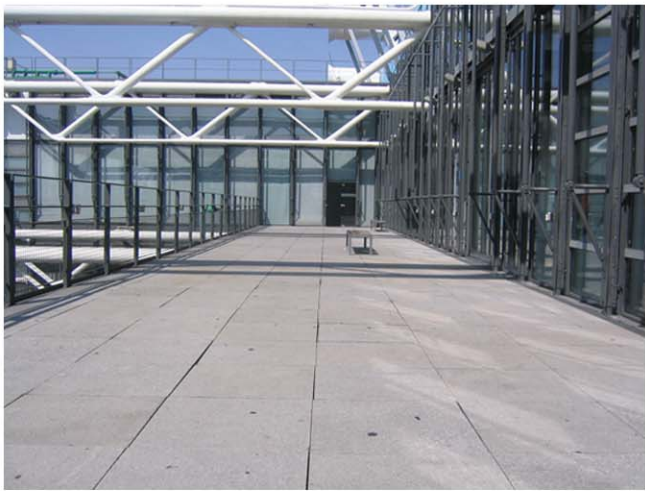
6th floor terrace
