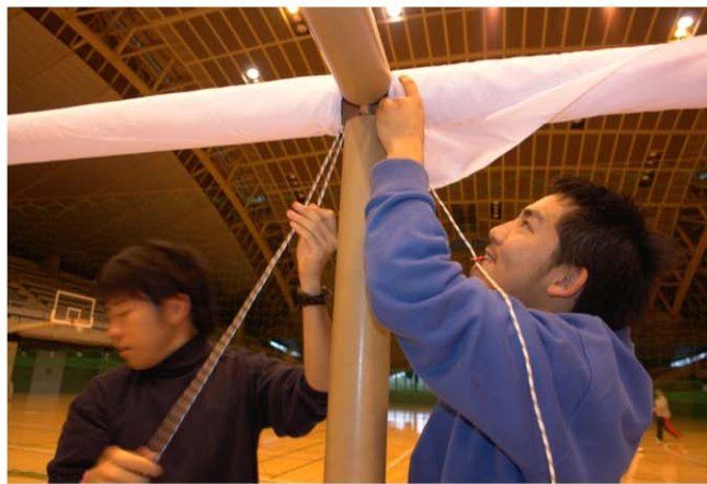
cross bracing with rope
