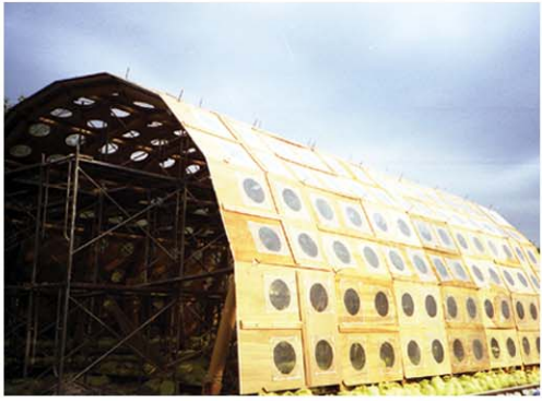
plywoods for the lateral stability
