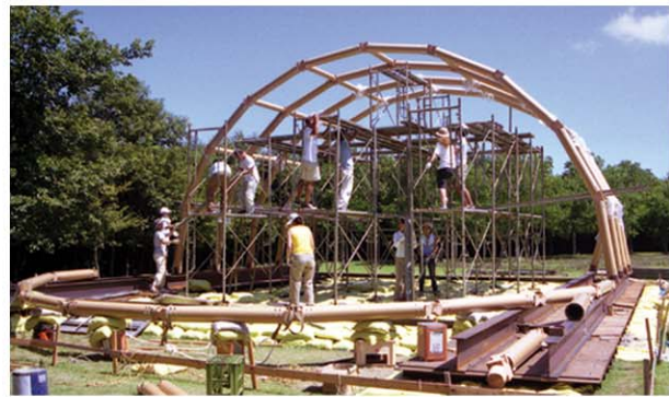
construction of the arches
