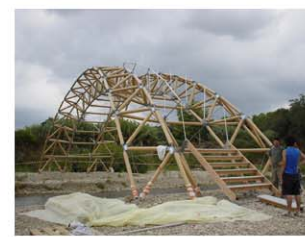
steps and handrails
