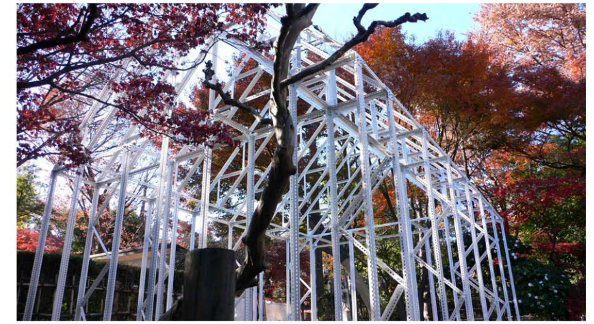
office-use steel shelf system as the main structural system
