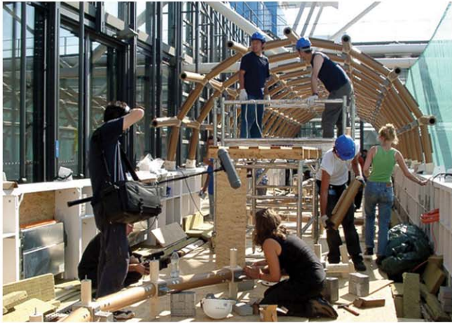
construction of the arches
