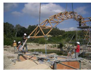
assembling on site
