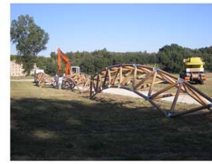
ready for transport
